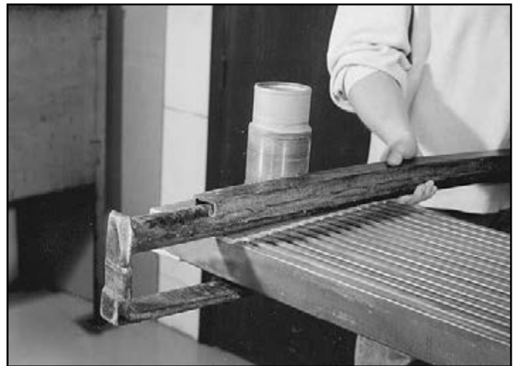
FIG. 25 Locate twisting hook as close as possible to the nozzle or stud
